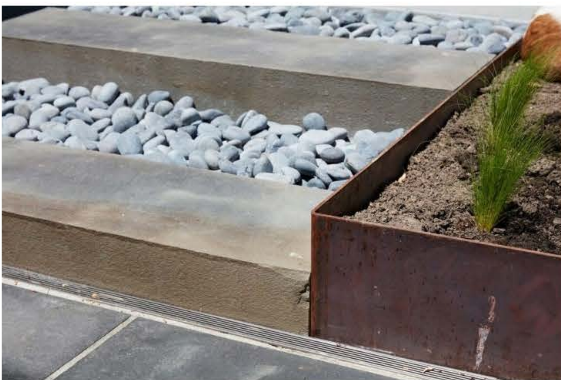
Above: A set of bluestone and river rock steps connects the two levels of the patio. For continuity, Choe used the same bluestone from the upper patio; the rocks are La Paz beach pebbles . At right: the corner of the Cor-ten steel garden bed. (For more, see Landscaping Ideas: 8 Surprising Ways to Use Cor-ten Steel in a Garden .)
